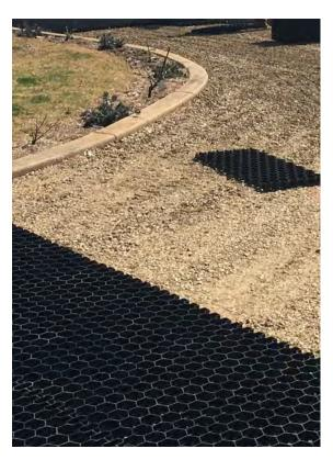
Step 3. Once the drainage base has been lightly compacted, start laying the GEOHEX™ pavers. When laying GEOHEX™, be sure that the male lugs are facing towards the outer edges of the install. This ensures the next piece you lay aligns the male lugs and female joints.
